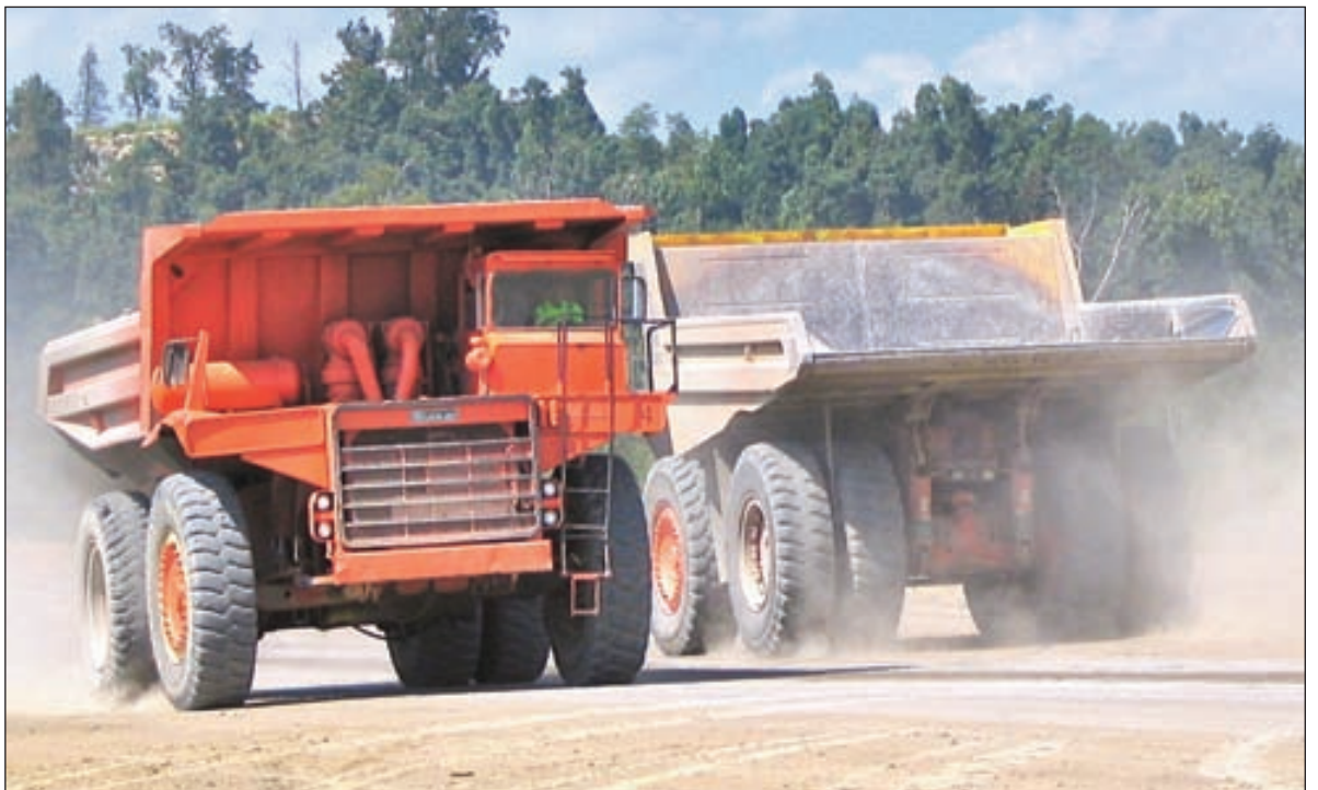
Two heavy earth-moving dump trucks meet one another last week on the road bed of the new U.S. 641 under construction in Crittenden County. The grade and drain phase of construction currently under way on the corridor-relocation project is expected to be complete before the end of 2014.
